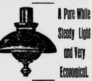
Consumes three (8) feet of gas per hour and gives an efficiency of sixty (80) candles. Saving at least 33<sup>1</sup> per cent. over the ordinary Tip Burners.
