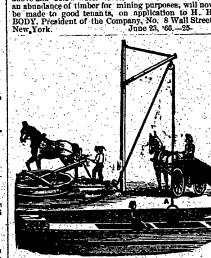
DEDERICK'S COAL HOISTING MACHINE, Patented April 12, 1862. This celebrated and unequalled Coal Hoisting Machine has been in successful operation for over three years, and the unusually large number already sold are giving the most perfect satisfaction. It is simple and durable, having no gearing at all; is rapid in its operation; and very easy for the horse. Descriptive Circular, containing letters of commendation, prices, &c., sent free, on spollcation. sent free, on application.
