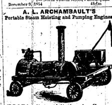
POR loading and discharging Cargoes, WOOD OR COAL CAN BE USED FOR FUEL.
