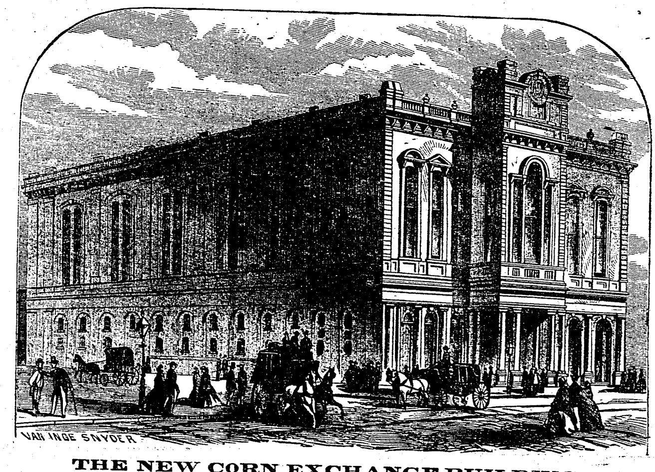
THE NEW CORN EXCHANGE BUILDING.
