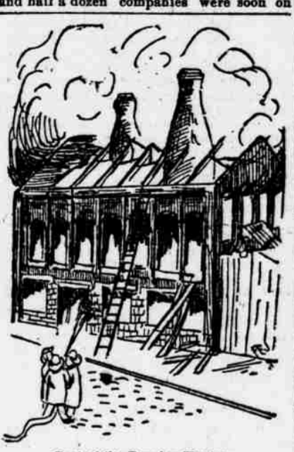
Part of the burning factory. The scene. Considerable delay in getting enough water gave the fire still better headway and all the buildings were in flames in an exceptionally brief time.
