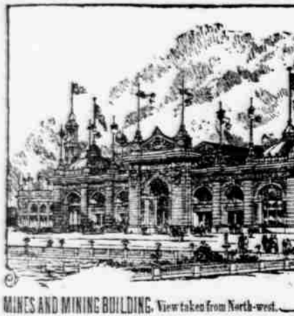
MINES AND MINING BUILDING. View taken from North-west.
