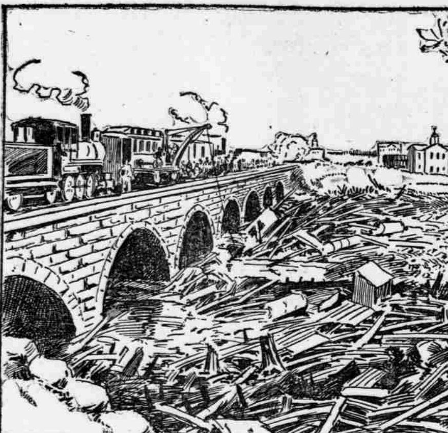
RAILROAD WRECKAGE ABOVE THE STONE BRIDGE. [Sketches by THE DISPATCH Artist Saturday, June 1, 1889.]
