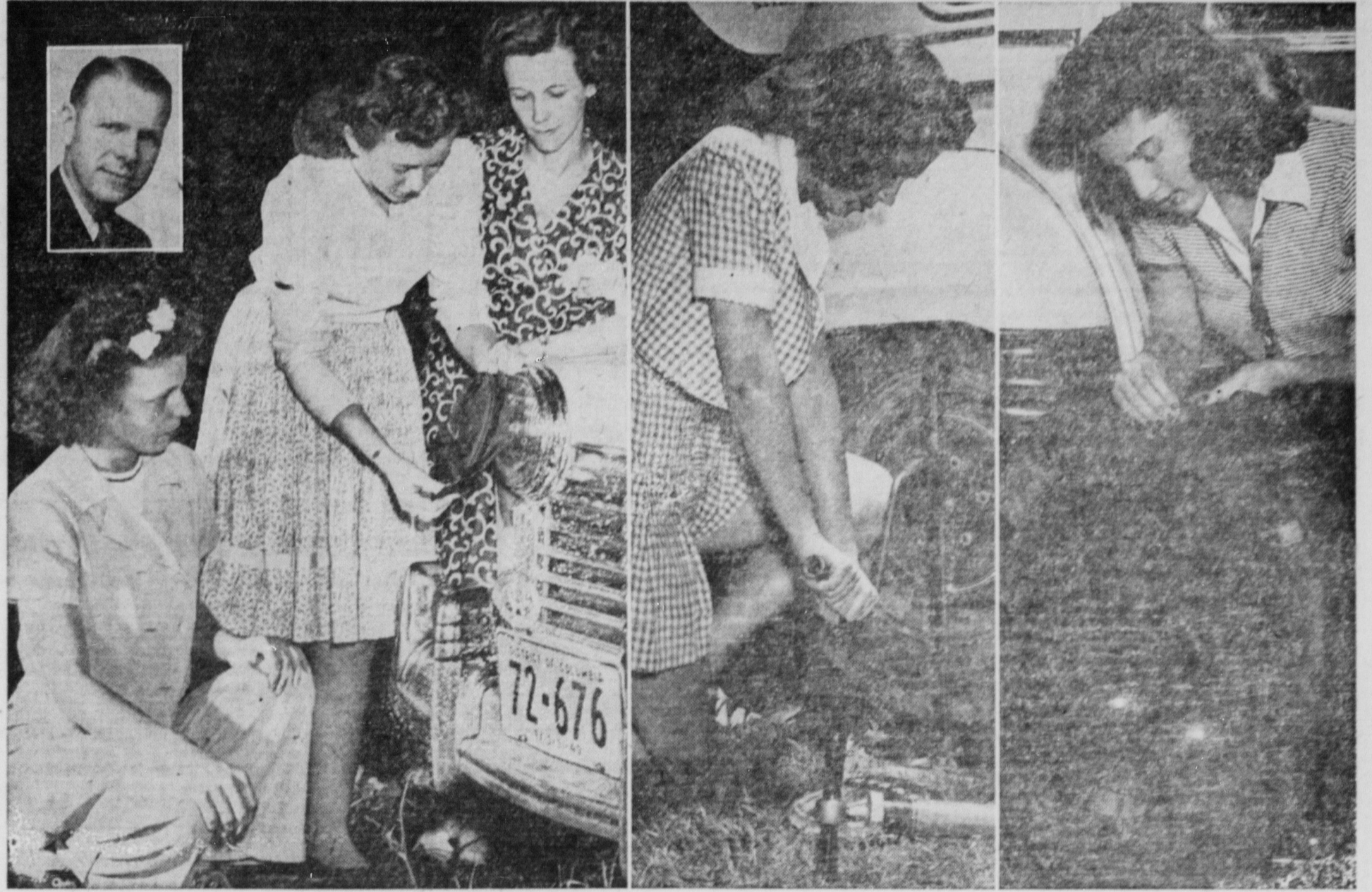
A blackout driving course, which has since been conducted elsewhere in the State and Nation by Prof. Amos E. Neyhart (inset), was first offered to members of the Drivers' Corps in Centre County. The scenes above, showing the application of a blackout mask (left), the removal of a tire (center), and the repair of an intertube, were typical of the course offered in State College last summer. In this and suc-
