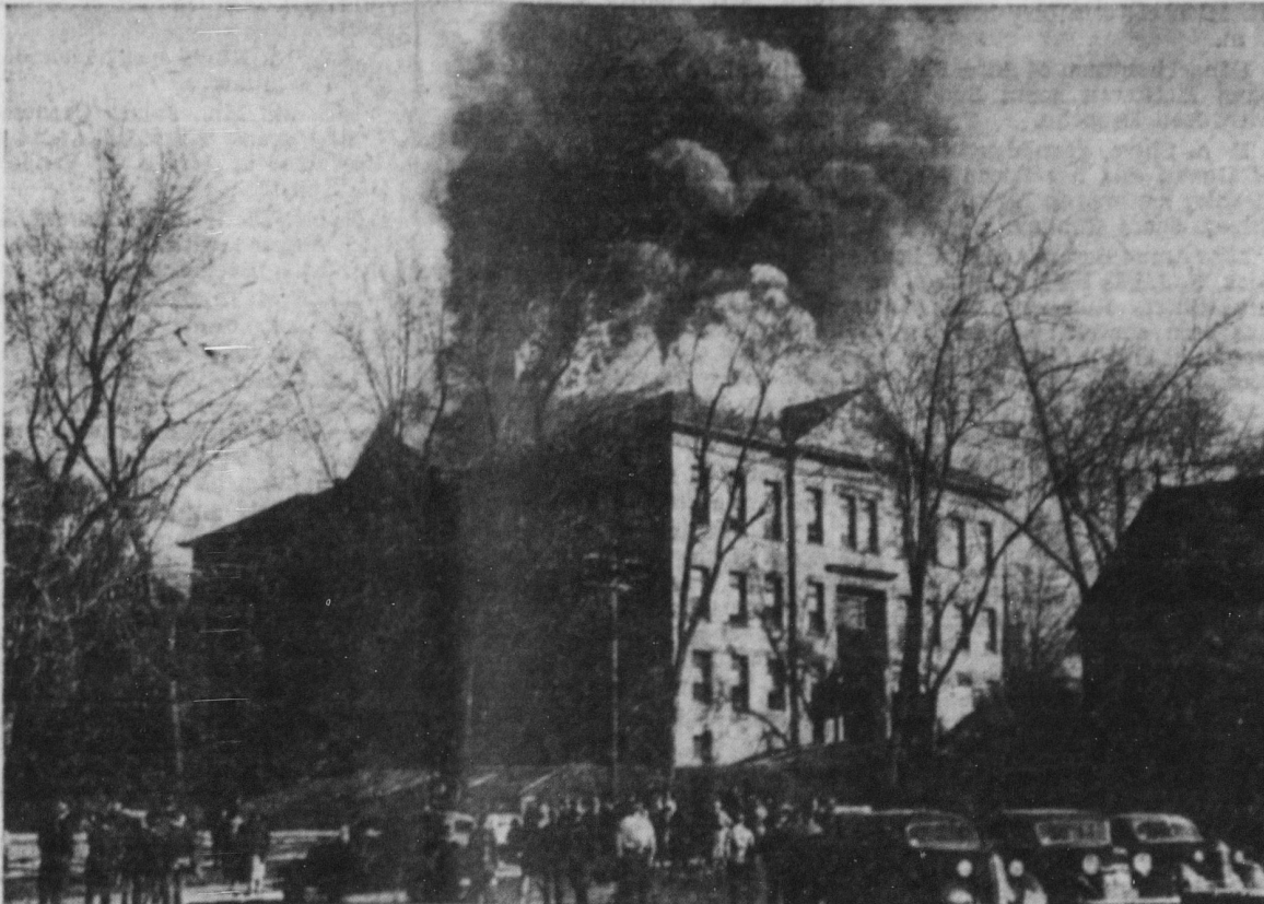
This photo, snapped not more than 10 minutes after the first flame broke through the roof, gives some idea of the speed with which the fire spread. View was taken from the old gas works site, on West Lamb Street.
