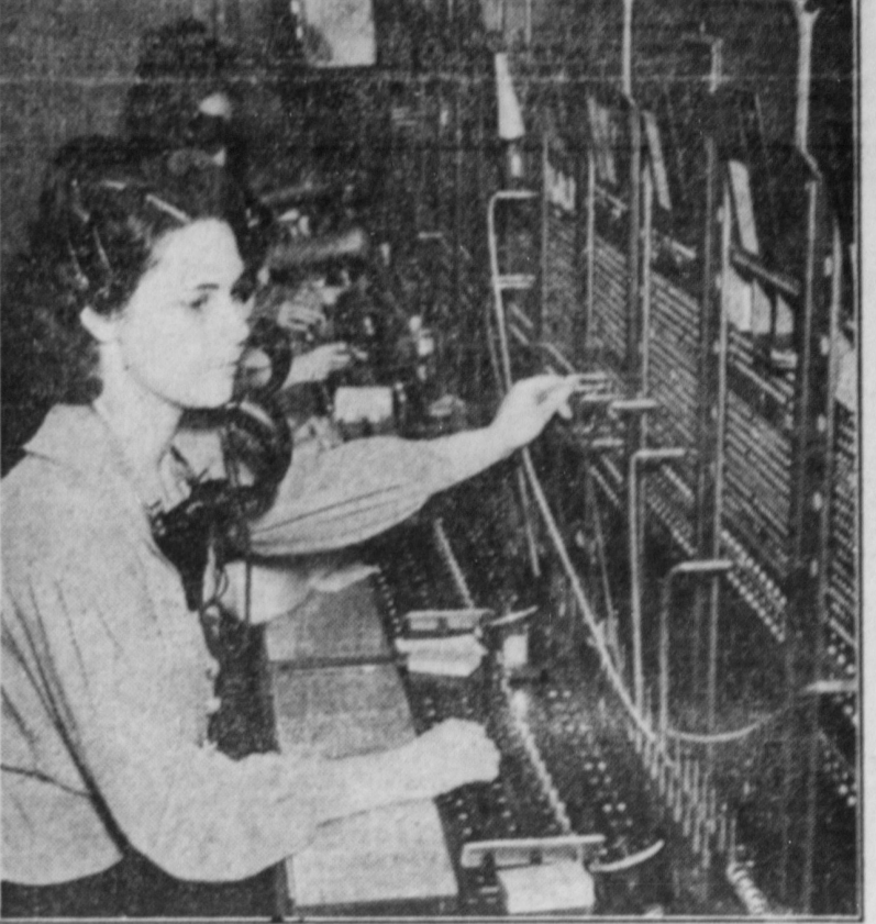
Twenty operators handle Bellefonte's 7,000 telephone calls originating here daily. Here is a picture of the telephone switchboard at 132 West High street, with Miss Louise Kline in the foreground. The Bell Company is holding an open house program this week at its central office, affording residents of this community an opportunity to see the switchboard and other intricate equipment in operation.
