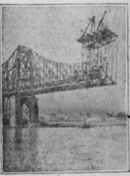
BLACKWELL'S ISLAND BRIDGE AS IT LOOKS NOW.
