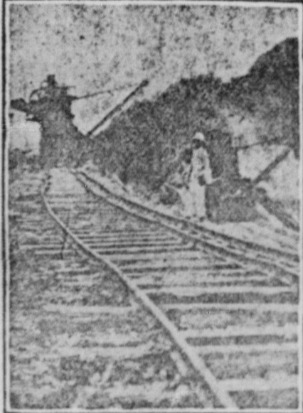
EXCAVATING WORK AT THE CULEBRA CUT.
