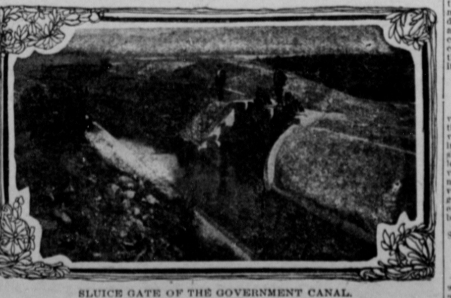
SLUICE GATE OF THE GOVERNMENT CANAL.
