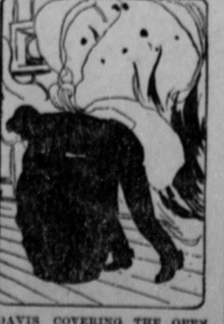
DAVIS COVERING THE OPEN POWDER BARREL FROM FIRE.
