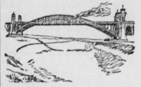
BRIDGE OVER THE CANAL AT GRUENTHAL.
