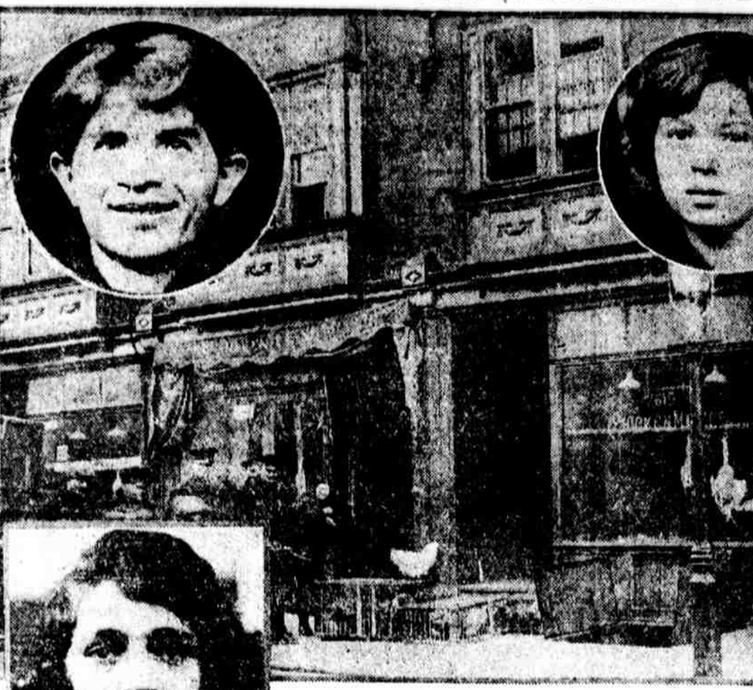
In center of upper picture are the houses, 2313 and 2315 South Seventh street, where eleven occupants were overcome by gas from a leaking street main. At right is Bertha Silverman, one of the victims, now in the Methodist Hospital, while at left is Harry Robbins, 2304 South Seventh street, who told Miss Sarah Lieberman, 2302 South Seventh street, about the drop, gave the alarm and aided in rescuing those overcome.
