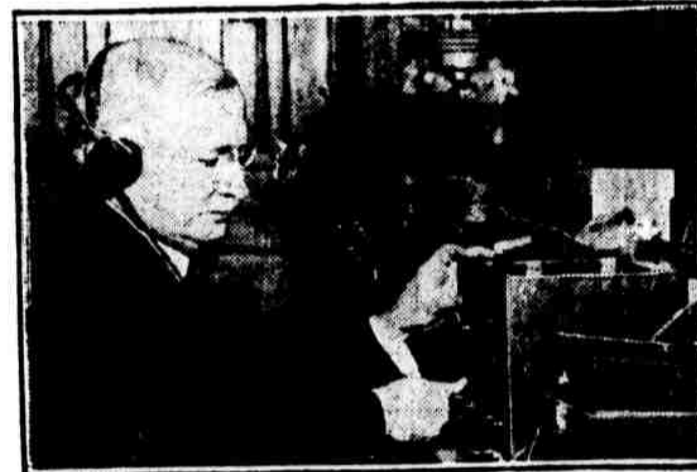
A PEEP INTO THE ELECTRICAL BUREAU at City Hall disclosed Chief McLaughlin busily experimenting with a wicked-looking radio outfit, which has recently been installed
