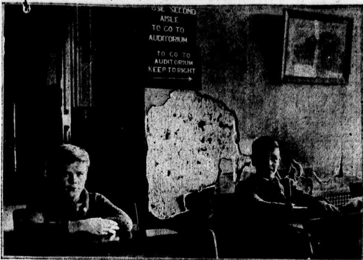
In this school, at Forty-first and Brown streets, the rooms are so overcrowded that five different classes must be accommodated each day in two rooms. Dilapidated condition of the school is considered a grave danger to pupils
