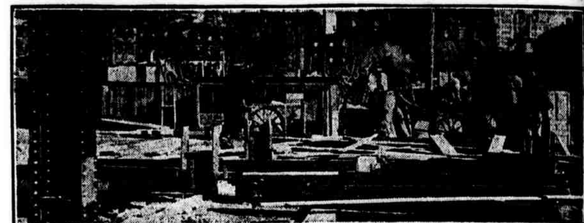
RAPID PROGRESS IS BEING MADE by the workmen engaged in construction of the new Philadelphia Free Library at Nineteenth and the Parkway. The work of putting in forms for re-reinforced concrete is shown above
