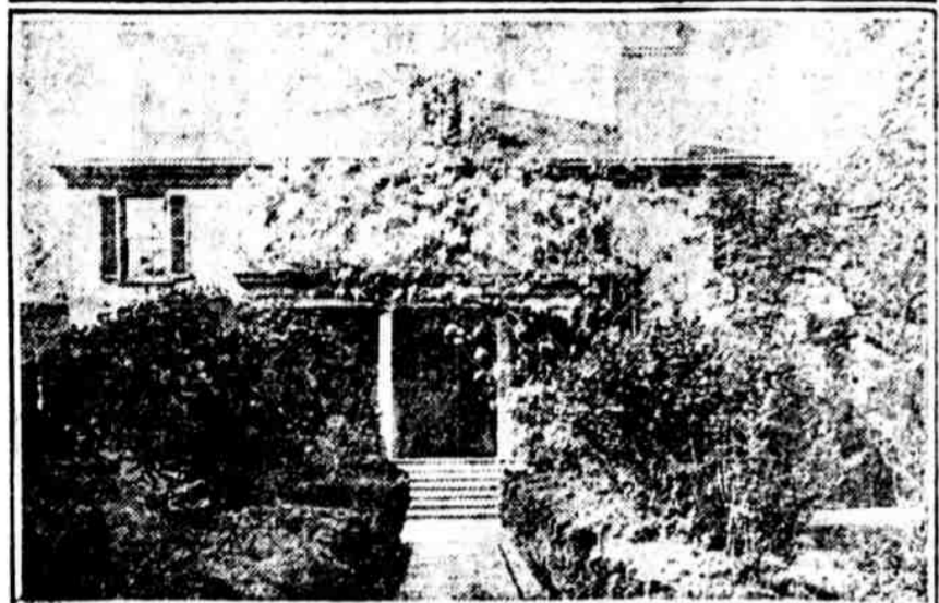
HOME OF THE LATE CHANDLER PRICE, as it looked on the north-west corner of Thirty-eighth and Chestnut streets, thirty years ago. An apartment house now covers the site. Linden T. Harris is the contributor
