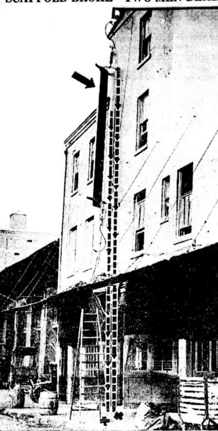
Two men were killed when a scaffold broke and fell from the side of a building under construction at Water and Dock streets.
