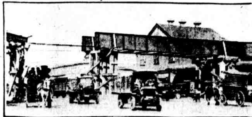
BRIDGING DELAWARE AVENUE. Over this bridge the equipment and material for the Delaware River Bridge will be handled
