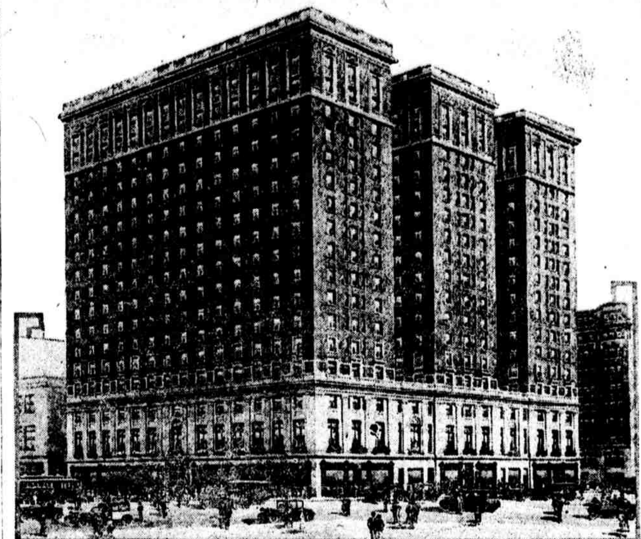
Plans are near completion for the building of this hotel, which is to rise on the site now occupied by the old Continental, at Ninth and Chestnut streets. Large subscriptions have been made by substantial men, and more are coming in. The architect is Horace K. Trumbauer.
