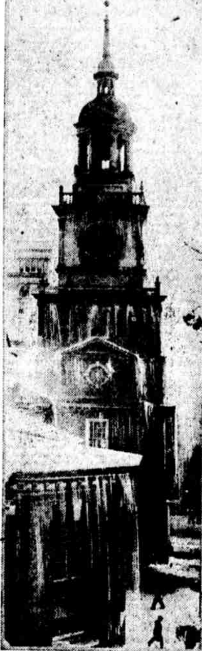
CURTAIN OF WATER City officials witness test of new sprinkler system designed to minimize fire danger at Independence Hall group
