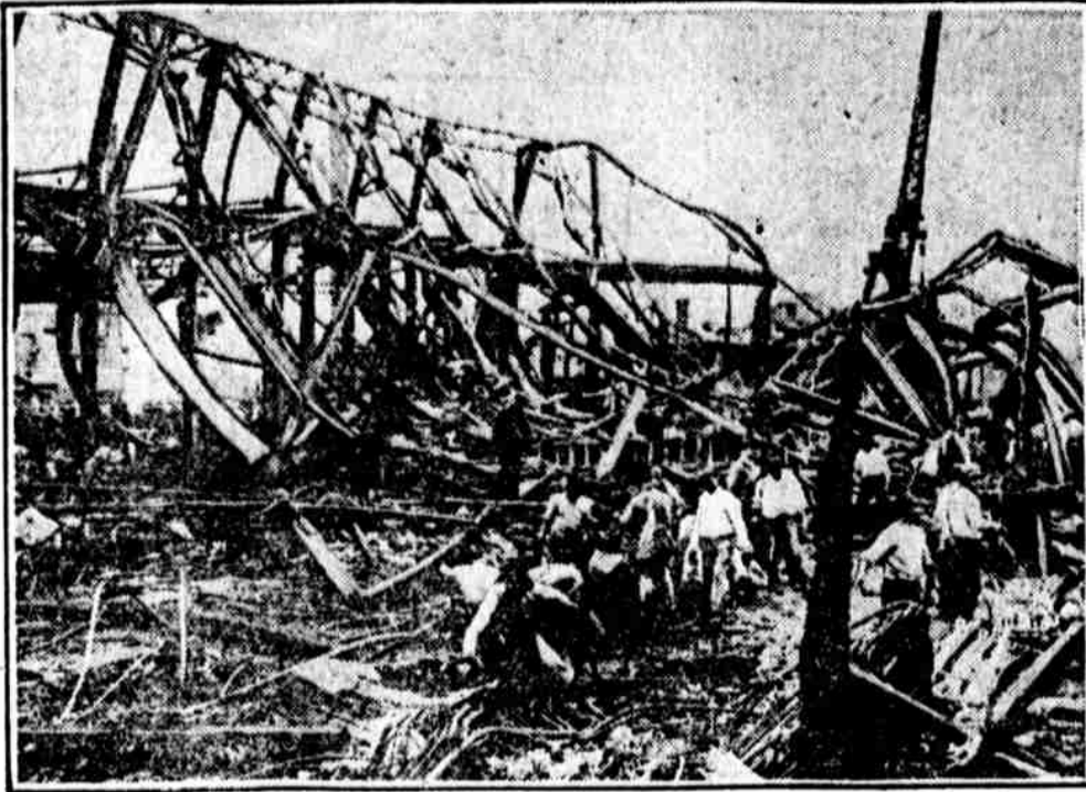
WHERE SEVEN RAILROAD SHOPMEN WERE BURNED TO DEATH. Ruins of the Pennsylvania Railroad's Thirteenth street barnhouse at Pittsburgh, where shop workers slept. Firemen are searching the ruins for other bodies
