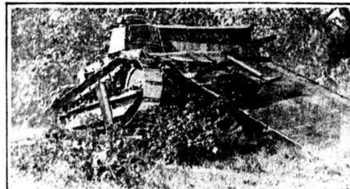
A WHIPPET TANK DEMOLISHES ARMY BUILDING
