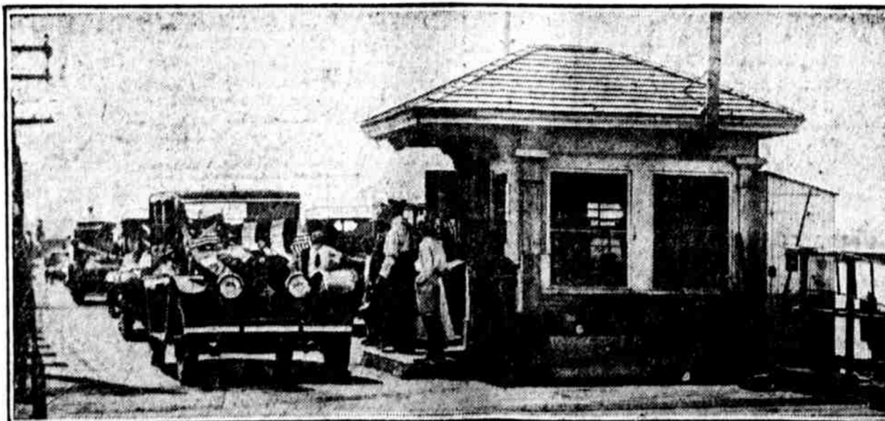
TOLL BRIDGE GOES—SHORE FOLK CELEBRATE. The bridge that connects Ocean City with Somers Point and Atlantic City is free, dating from yesterday. Officials of shore towns were in the first cars that crossed the bridge in its free state
