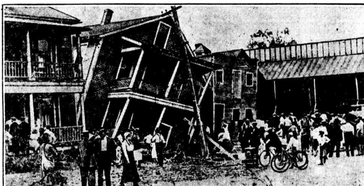
$1,000,000 PROPERTY LOSS WHEN DAMS BURST AND FLOOD MASSACHUSETTS TOWN. Twenty million gallons of water flooded the Williamsett section of Chicopee, Mass., early Monday morning as a result of the bursting of two dams. Photograph shows a wrecked house, the occupants of which had a narrow escape from death. They escaped by means of a plank laid from a second-floor window to the house next door
