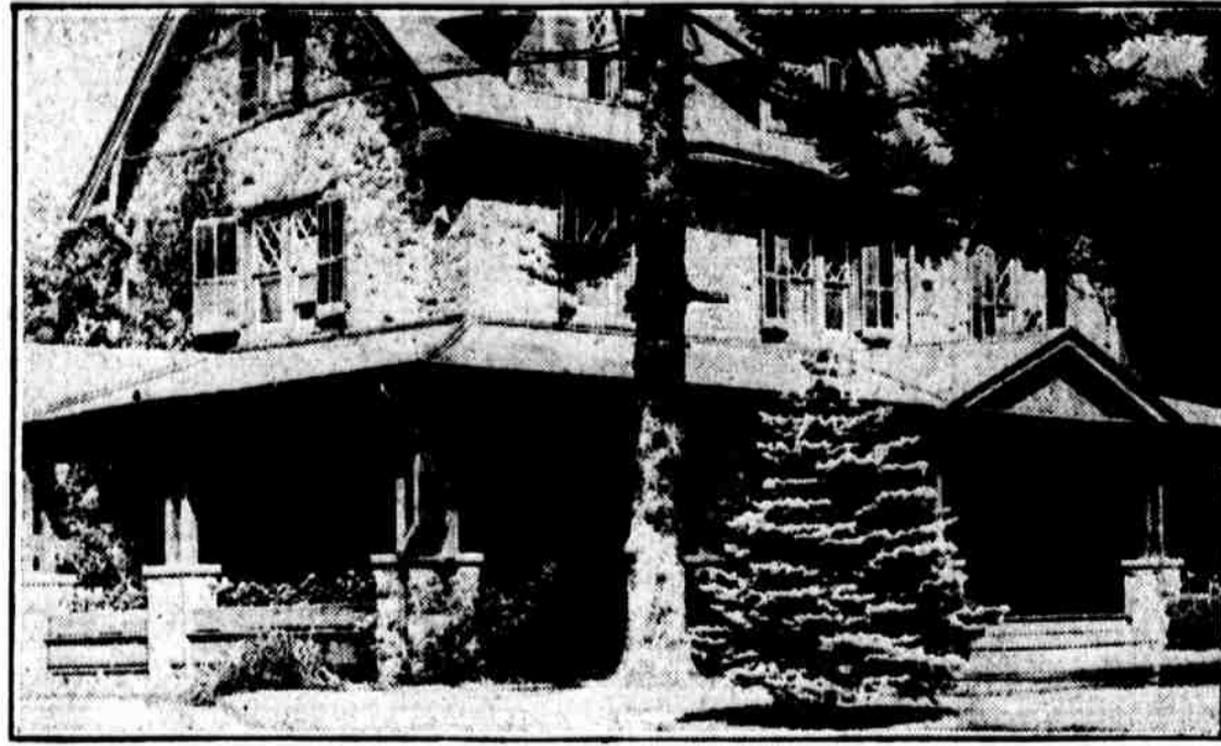
THE BRINTONS' SUMMER HOME. It is at Rosemont and is the property of Eckley B. Cox. The police found the house on fire, and were forced to go through the smoke to the third floor before taking their prisoner
