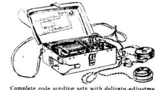
Complete code sending sets with delicate adjustments to insure perfect signals. Packed in rolled steel boxes covered with heavy leather, with carrying strap, bronze buckles and trimmings.
