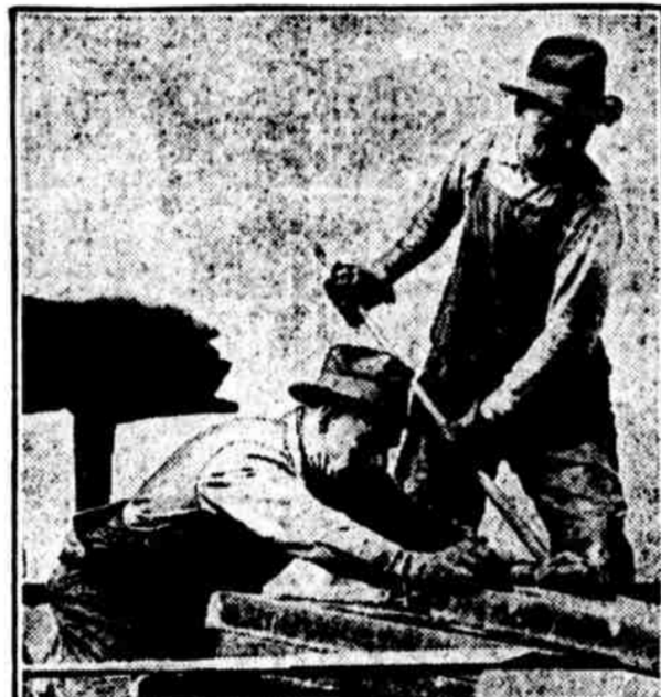
AIDING IN ERECTION OF PHILADELPHIA LIBRARY. Hector McQuarrie (left), and Charles Masdow, handling 500-pound steel slabs
