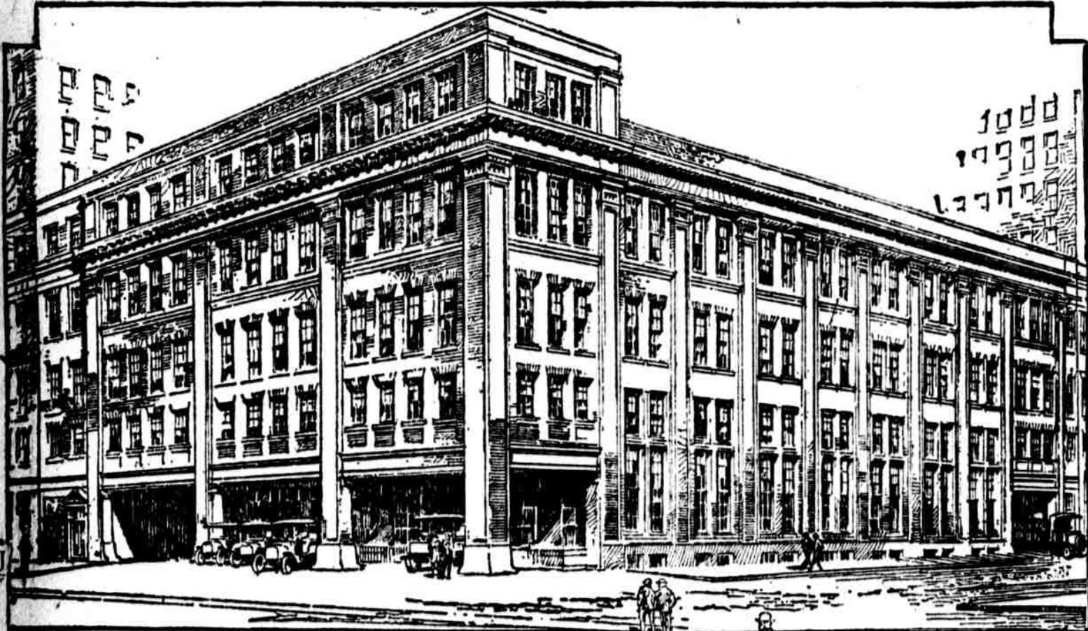
THE FIRST UNIT IN THE NEW HOME OF THE PUBLIC LEDGER COMPANY. This great new printing plant, when completed at a cost of $1,250,000, will house the most modern press and auxiliary press equipment, valued at approximately the same amount. The site, at the northeast corner of Seventh and Sansom streets (above) will soon be ready for the builders. The first brick was taken from the old buildings at Seventh and Sansom streets on March 10 of this year. Apart from its own importance, this new building is of interest because it is the first unit in the PUBLIC LEDGER'S new home, which will cover the whole block between Sixth and Seventh streets and Chestnut and Sansom streets. Construction of the two other units, ten stories high, will start soon
