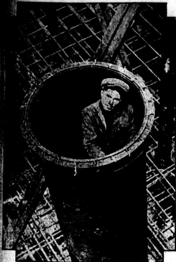
CLOSE-UP OF THE DELAWARE RIVER CAISSON. Ralph Terranova, a compressed air expert, posed in one of the muck locks, through which mud will be removed from the bed of the river. Over at the right is one of the chutes that will carry cement down into the huge steel box.
