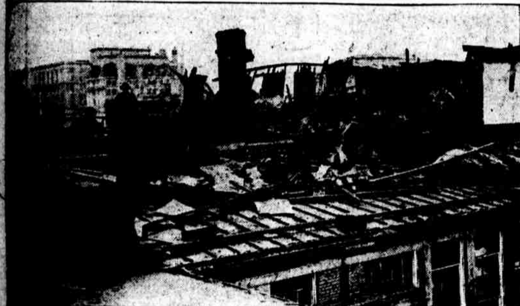
TREASURY DEPARTMENT BUILDING HAS ANOTHER MYSTERIOUS FIRE. For the second time in three months Washington firemen were called out in the wee hours of the morning to fight a blaze of unknown origin on the roof H. & F.
