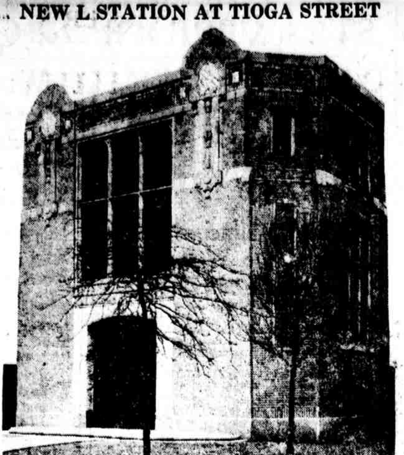
NEW L STATION AT TIOGA STREET This station stands at entrance to Harrowgate Park. There is an arcade through the building from the street to the park. The station is of brick with buff tapestry, terra-cotta trimmings and marble inserts
