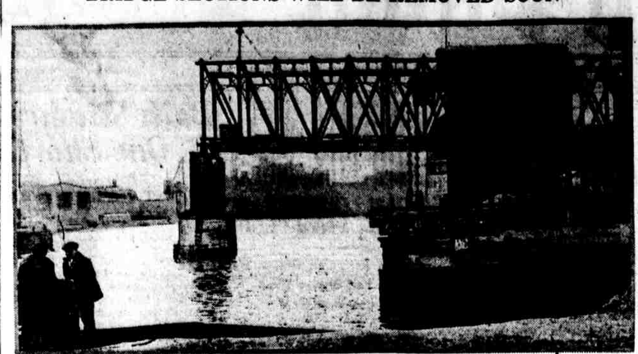
The first section, weighing about 900 tons, will be taken from the South Street Bridge piers in a few days in one piece. The new bridge will be started as soon as the old one is cleared away.
