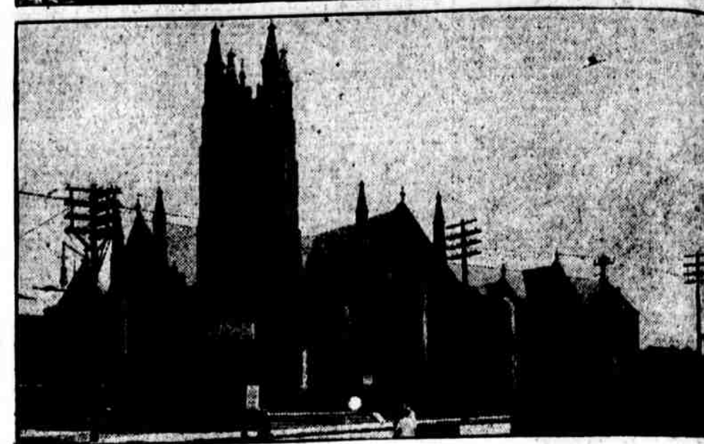
A MARVELOUS CHANGE IN SIXTEEN YEARS. The upper view shows how the northwest corner of Fifty-eighth street and Chester avenue looked in 1908. Below is the Westminster Presbyterian Church, which now occupies the site. The photographs were contributed by John W. Culbertson, 5641 Chester avenue. If you have old-Philadelphia photographs send them to the EVENING PUBLIC LEDGER
