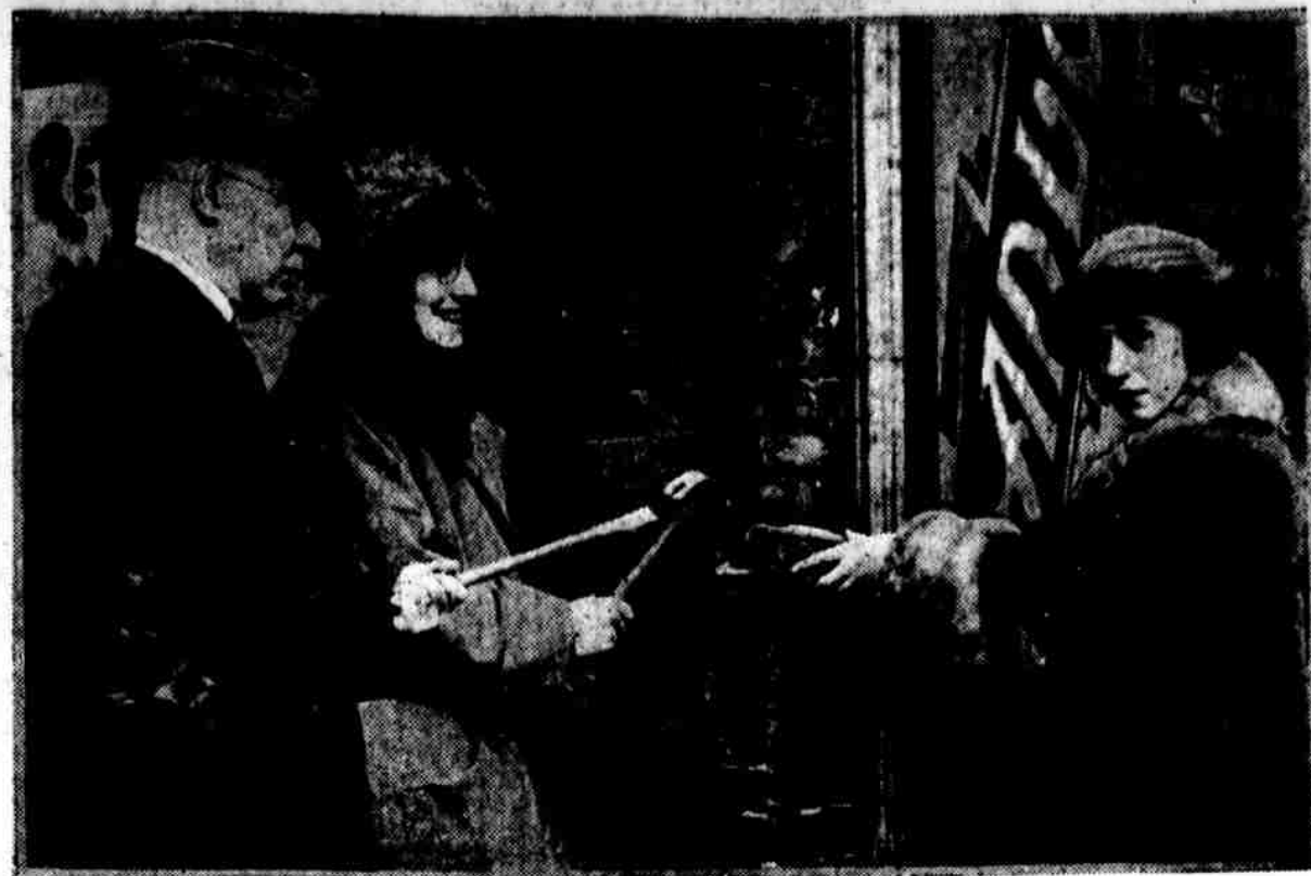
MAKE START ON CLEARING SITE This photograph was made this morning at the northeast corner of Seventh and Sansom streets, the first building to go in clearing the site for the new home of the Public Ledger, morning, evening and Sunday. Charles Reed, chief engineer of the Public Ledger Building; Mrs. Frieda Kipp and Miss Ethel Till, shown here in the order named, loosened the first bricks.
