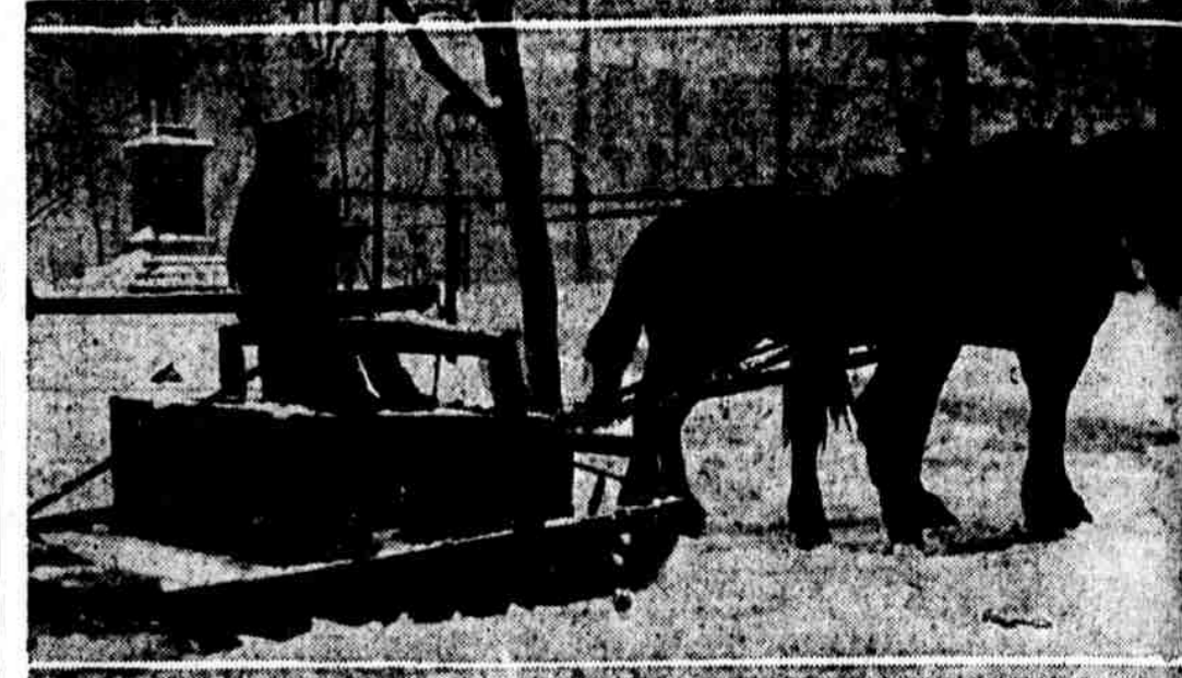
REMOVING SNOW FROM WALKS. This snow-clearing device was put into service in Independence Square yesterday morning by the Bureau of City Property
