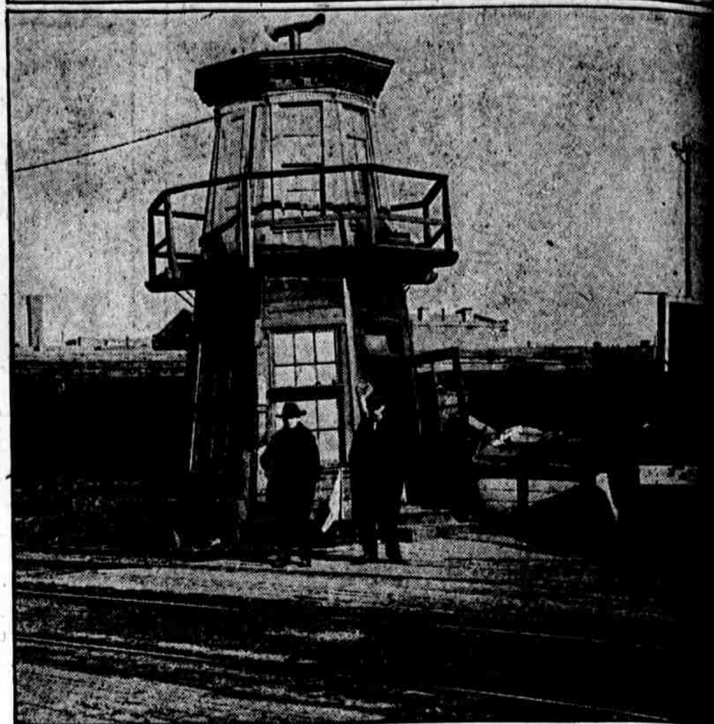
AN OLD PHILADELPHIA AND READING SIGNAL TOWER. It was at Tenth and Diamond streets and was the first tower used for signaling trains by that Company in Philadelphia. The photo was made by C. H. Miller, of 3215 North Park avenue, in 1886. Mr. Miller contributed the photograph. Have you an old-Philadelphia photograph? Send it to the EVENING PUBLIC LEDGER
