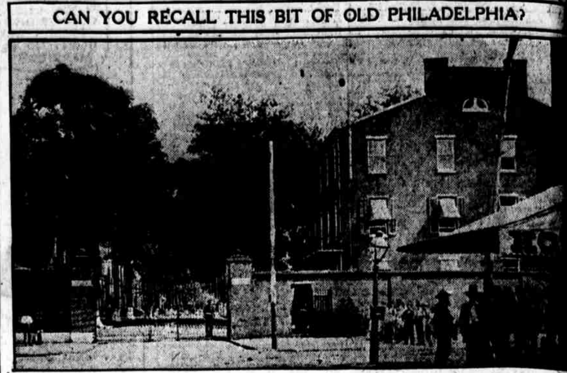
CAN YOU RECALL THIS BIT OF OLD PHILADELPHIA? WHERE A FORMER NAVY YARD WAS LOCATED. View of the entrance to the old Philadelphia Navy Yard, at Front and Federal streets. All naval work was done here until the League Island site was taken over by the Government. F. A. Fuhrmeister, Jr., of 2000 Emily street, contributed the photograph. Have you an old-Philadelphia photograph? Send it to the EVENING PUBLIC LEDGER
