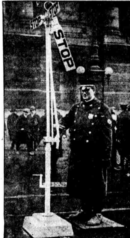
MUCH WHITE PAINT. Traffic semaphore at Juniper and Market streets is readily seen. The sentinel is Charles Rosenberger.
