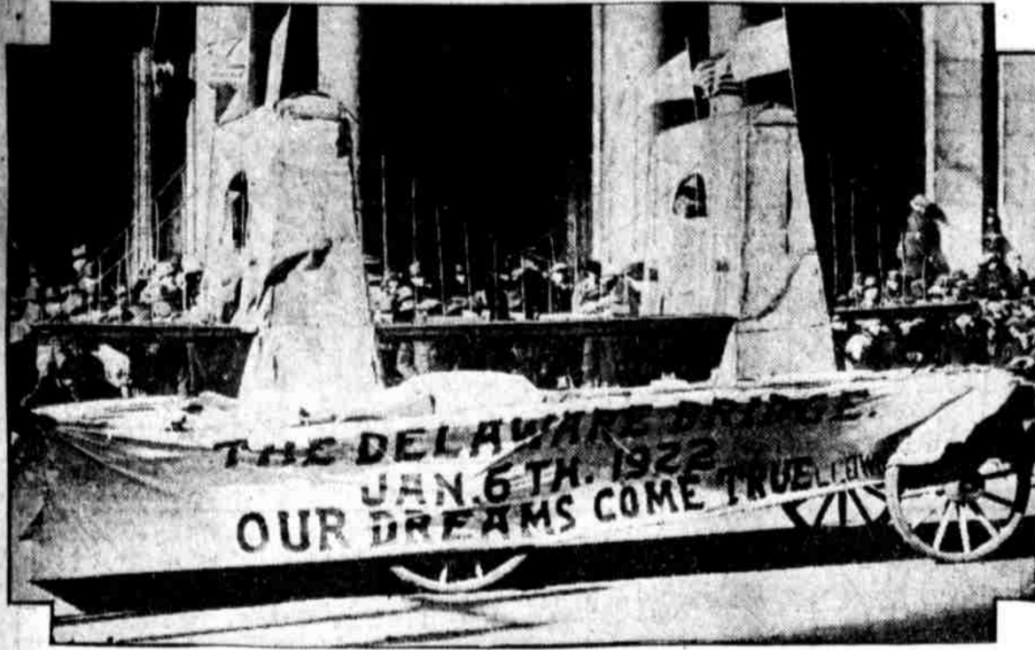
WON SECOND PRIZE FOR FLOATS. The Camden Clowns took $125 as a prize for this Delaware River Bridge float in yesterday's Mummers' parade. It was timely, due to the fact that ground will be broken this week for the long-hoped-for bridge.
