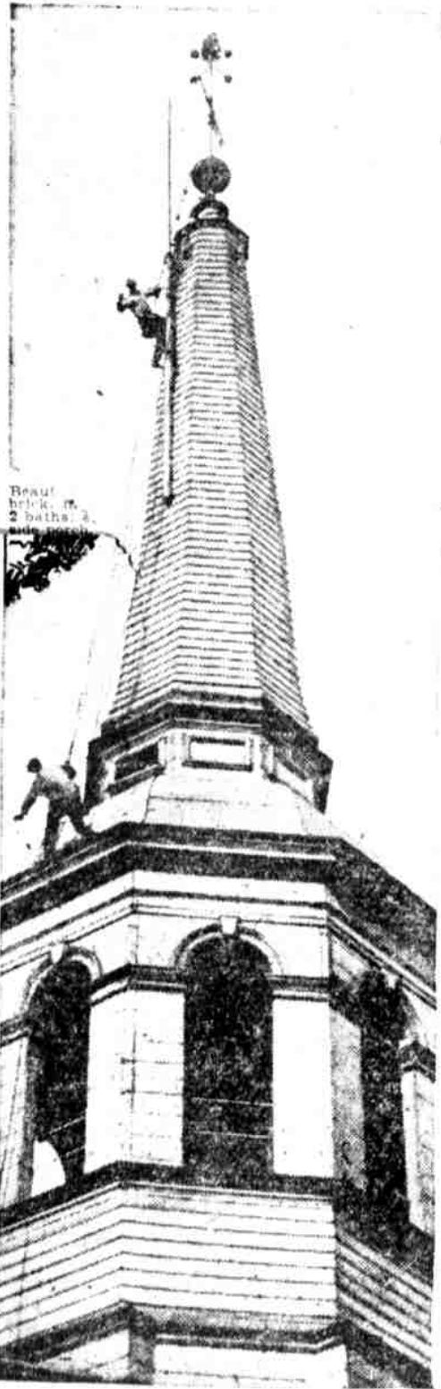
STEEPLEJACKS IN ACTION. Christ Church steeple is being repaired and painted.
