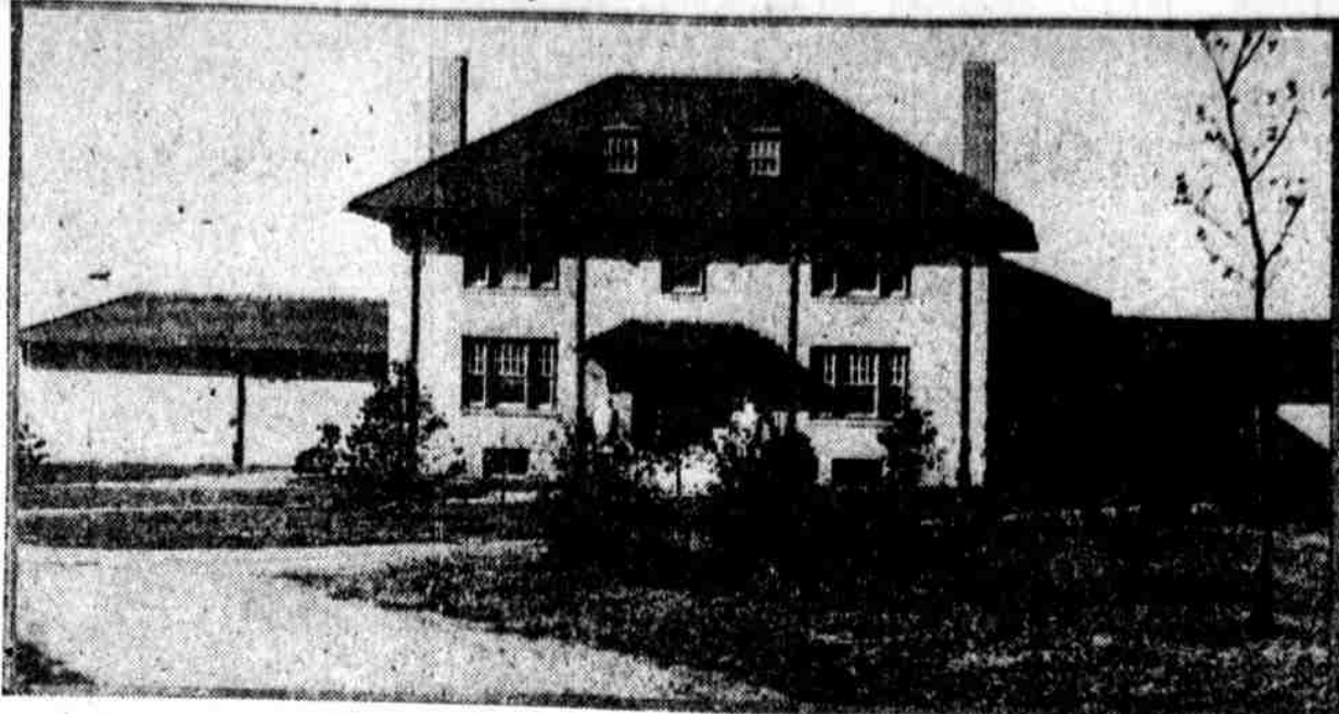
This $75,000 building, erected during the Smith-Vare Administration, on League Island Park, still is awaiting actual use.
