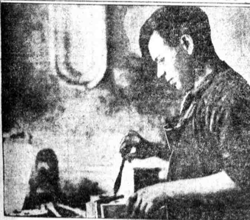
ABE PASTON, 5507 Lansdowne avenue, soldering lids on bread boxes in the factory of C. B. Porter Company, tinware manufacturers, 128 North Second street.
