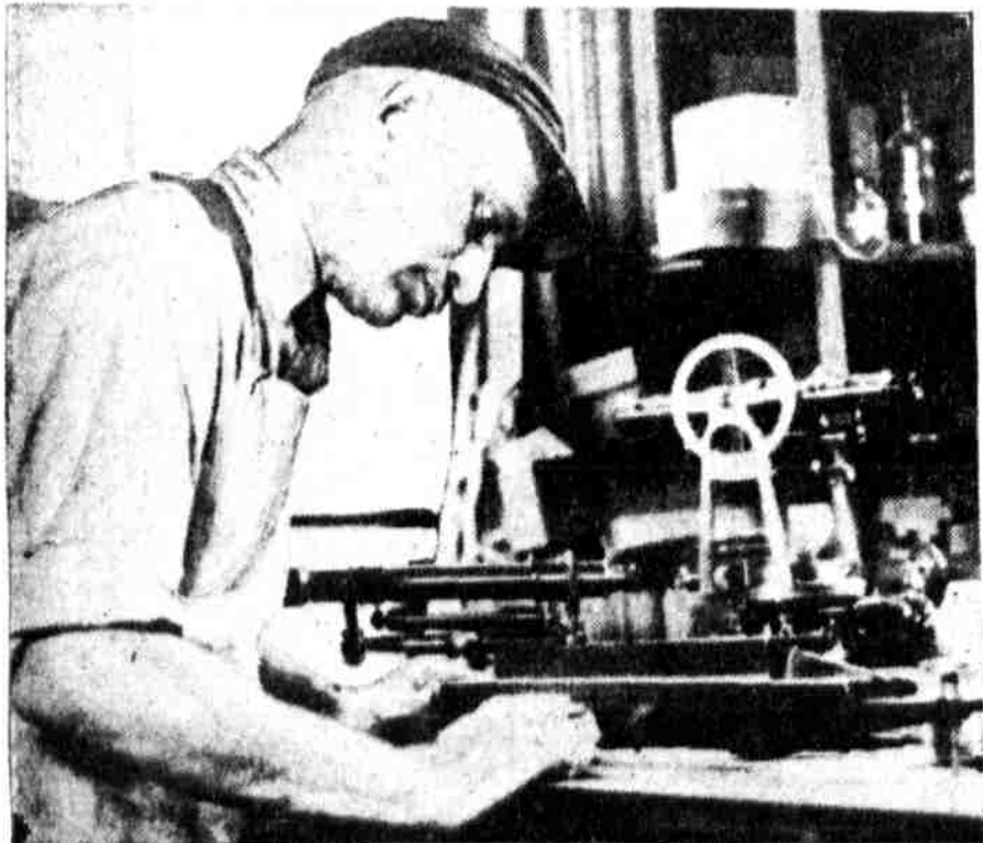
FINAL ADJUSTMENT. Frank M. Klotz, 6031 Magnolia avenue, working on precision levels, used for setting up intricate machinery. They're being made in the factory of Queen-Gray Company, 70 W. Johnson street. L. P. S.
