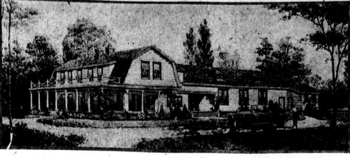
New Jersey grand officers to lay cornerstone of building, designed as social and recreational center
