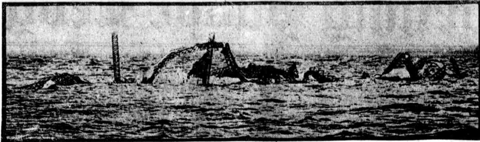
Above is shown a full-length picture of the shattered skeleton of the wrecked ZR-2 as the splintered and twisted framework of the erstwhile queen of the air was slowly sinking into the mire of the Humber River.
