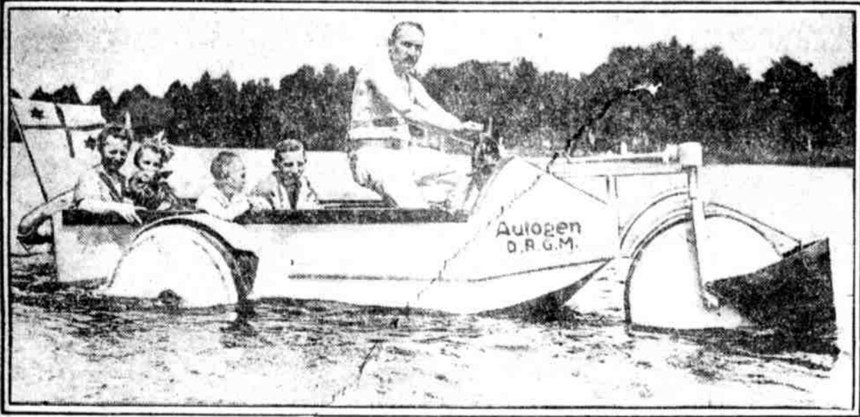
ON LAND OR SEA. This new wrinkle of transportation is being used in the waters of the Rhine. When it gets in water, the small paddle wheels attached to the road wheels are put into action.
